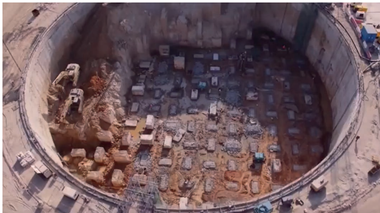
The Dubai Creek Harbour Tower - @DR
